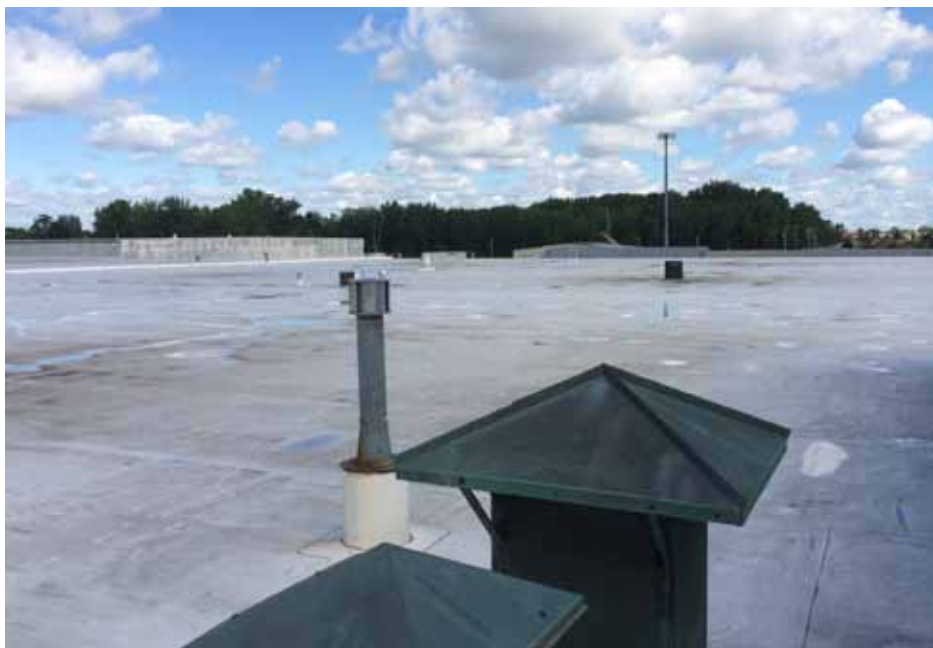
RAV Properties (Thompson Road, Syracuse) - Insulated TPO (Thermal Plastic) Roof, 140,000 Sq.Ft
